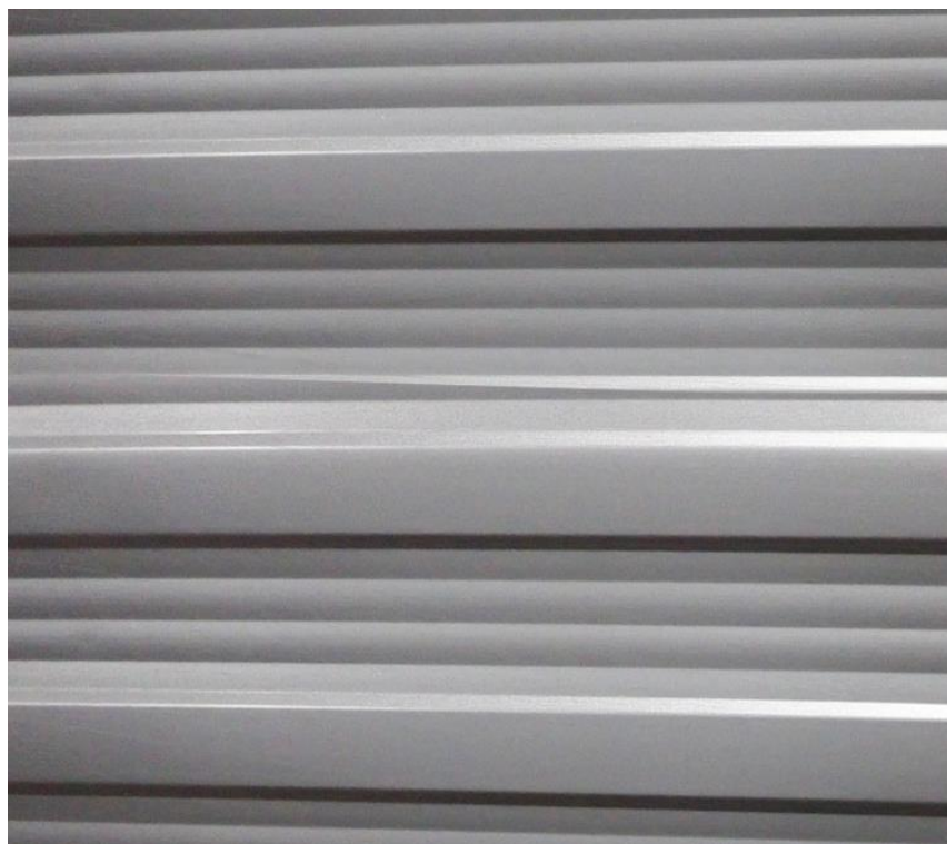
SILVER SPUR MESA EXTERIOR SIDING
